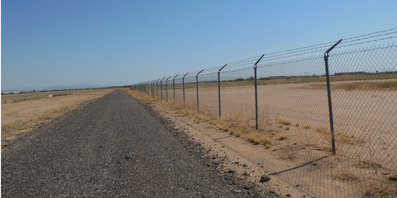
PERIMETER SERVICE ROAD AND SECURITY FENCING
