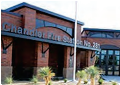
Station No. 1 1491 E Pecos Road
