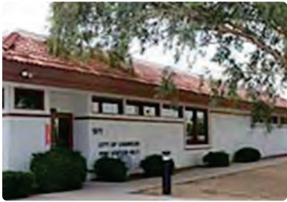
Station No. 4 295 N Kyrene Road
