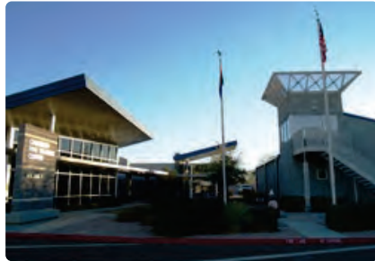
Fire Training Center 3550 S. Dobson Road
