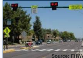
Pedestrian signal: flashing signal that stops traffic only when needed
