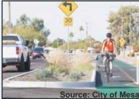
Separated bike lane: bike lane protected from roadway
