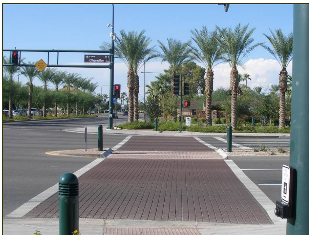
Figure 6-2: Refuge Island for Pedestrians and Bicyclists on a Busy Roadway
