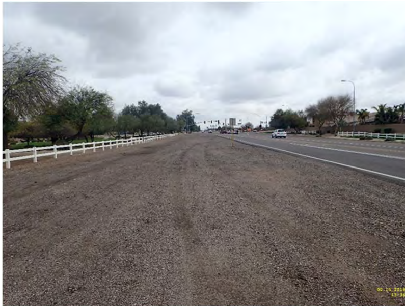
View from the western project limits at Kingston St. looking east along Chandler Heights Road.
