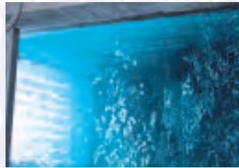
Ultra violet lights disinfect the wastewater
