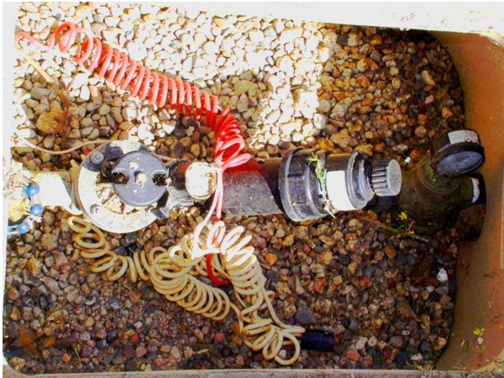
Be sure to check the wire connections. A very common irrigation system failure is when regular wire nuts are used. There is a high level of moisture inside of the boxes from condensation and corrosion on the wires will stop the valve from opening when the controller sends the signal. Use waterproof wire connectors. These can be as simple as wire nuts that are pre-filled with silicone.
