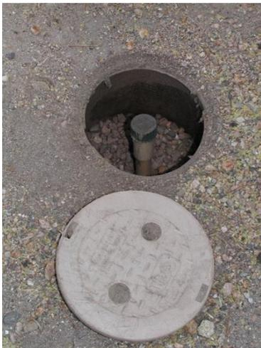
If your system has the threaded caps inside of pit boxes, unscrew the cap before turning the zone on. The water will be at a lower pressure and will fill the box with water. Just like the filters, they have hose threads, not pipe threads so use the short piece of garden hose to keep the box dry like with the filter flushing.
