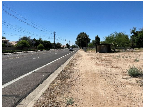
Figure 7 - Kyrene Road Missing Sidewalk
