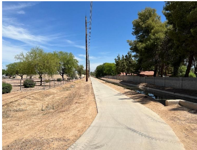
Figure 3 - Existing Kyrene Branch Canal Shared Use Path, Tempe
