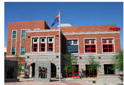
Chandler's Fire, Health, and Medical Department headquarters
