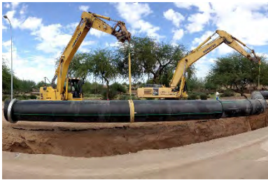
Infrastructure placement and upgrades
