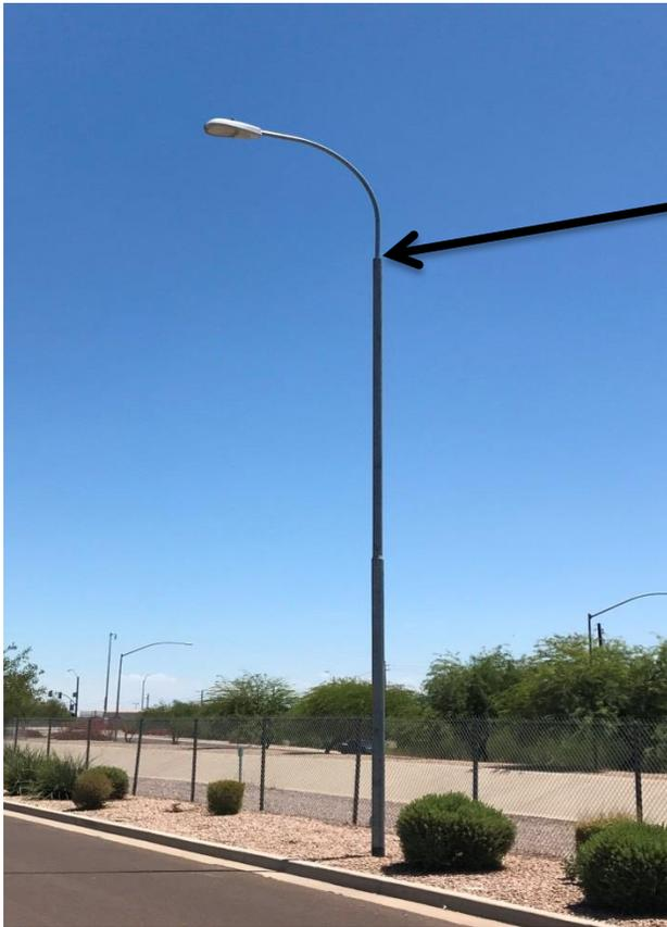
The "Connection Point" on an Existing Telescopic Style Streetlight Pole with an Integrated Luminaire Mast Arm
