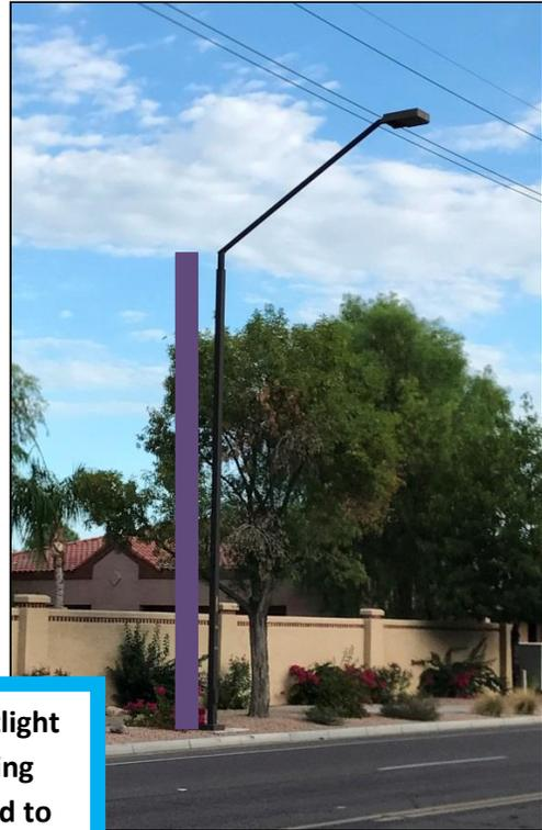
The purple line next to the streetlight depicts the section of the existing streetlight pole that shall be used to calculate the height of the existing pole. The lines are not to scale and are solely used for illustrative purposes.
