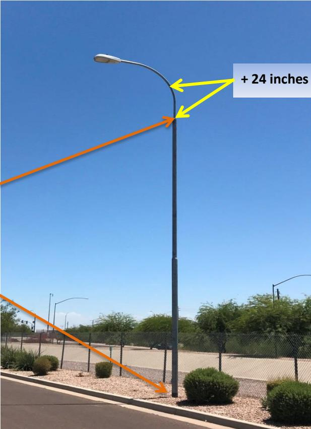
The Top and Bottom Points on a Telescopic Streetlight Pole to Calculate the Vertical Height of the Existing Streetlight Pole **PLUS** Twenty-four (24) inches
